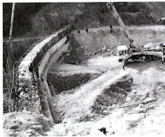
(d) HSCC casted by a pump truck
